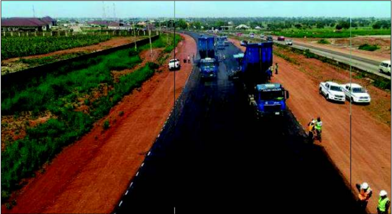
CONSTRUCTION OF THE OF THE ABUJA TO KANO ROAD
