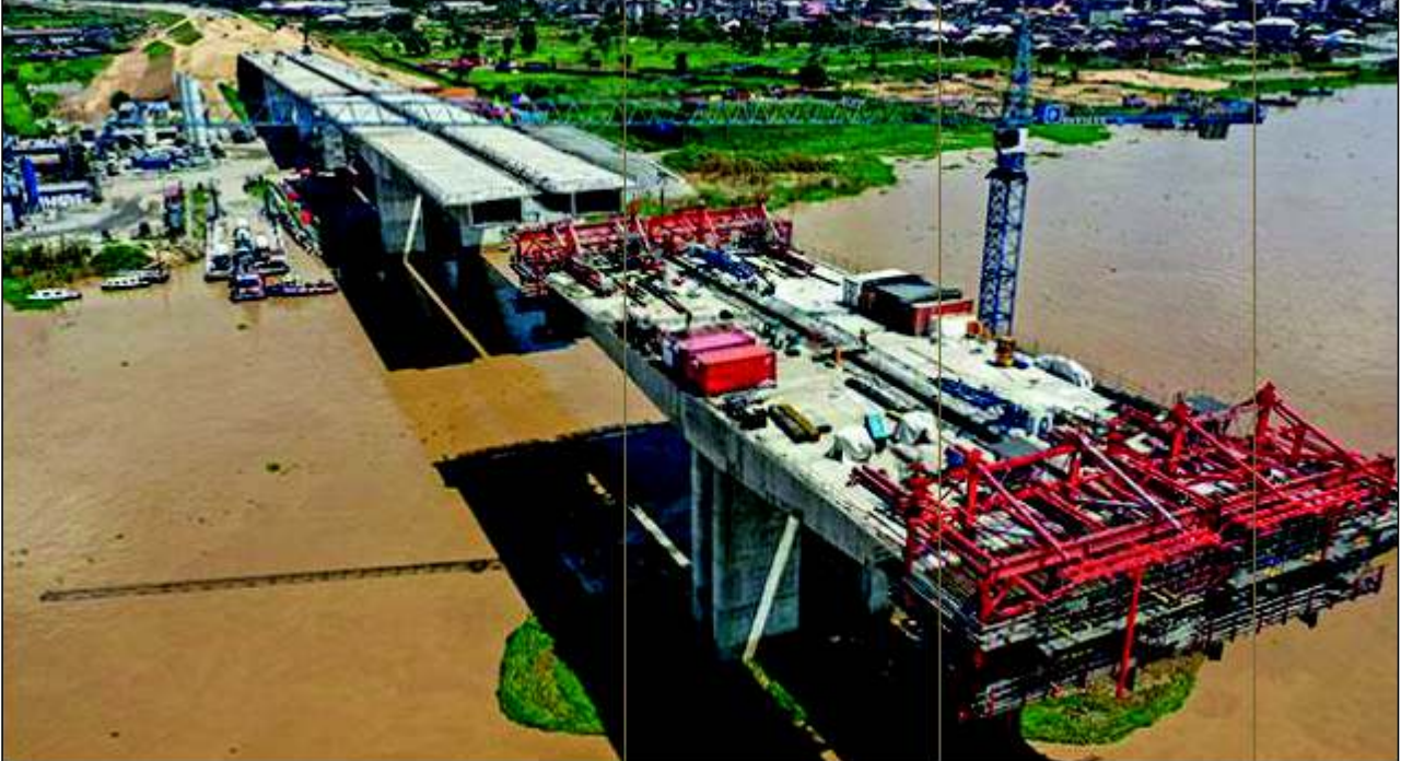
CONSTRUCTION OF THE SECOND NIGER BRIDGE
