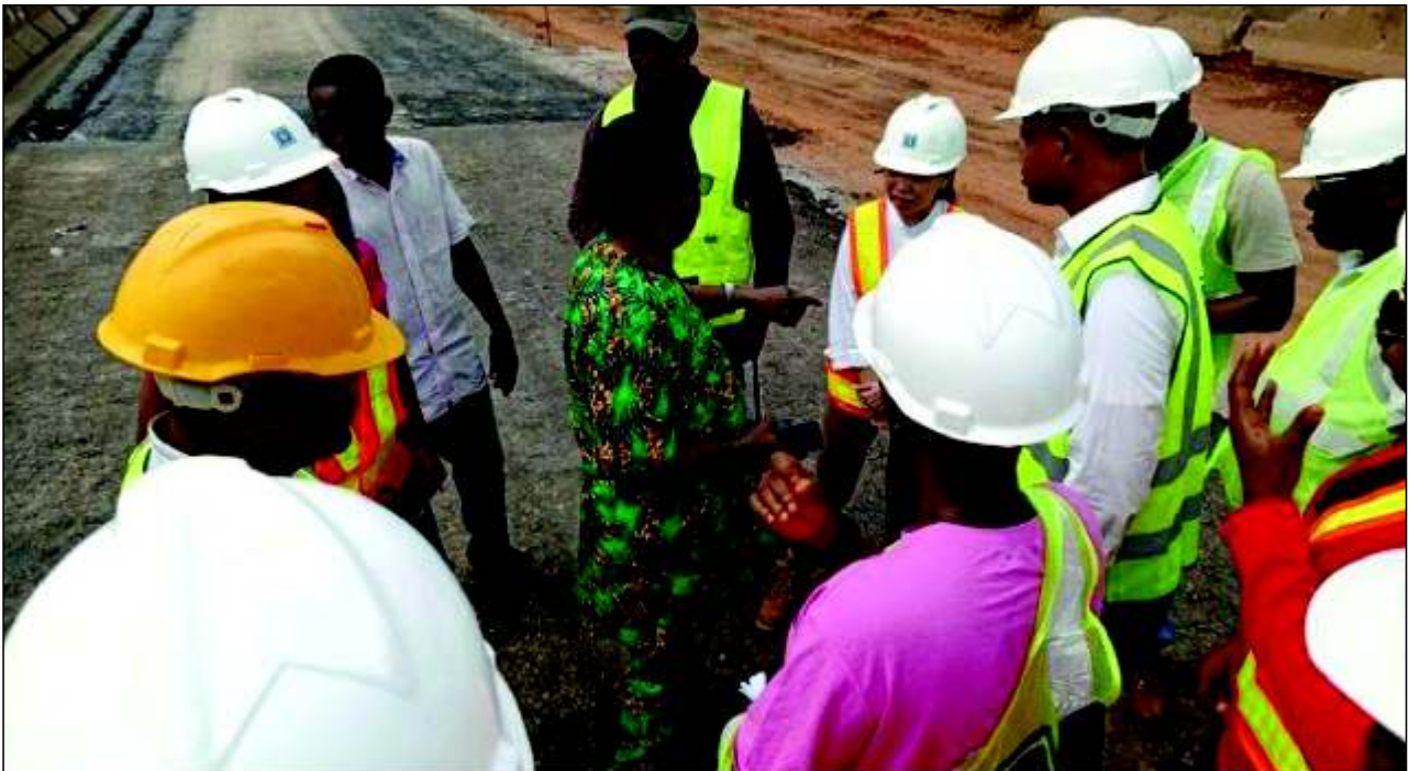
FIFTH MONITORING VISIT TO THE LAGOS/IBADAN ROAD
